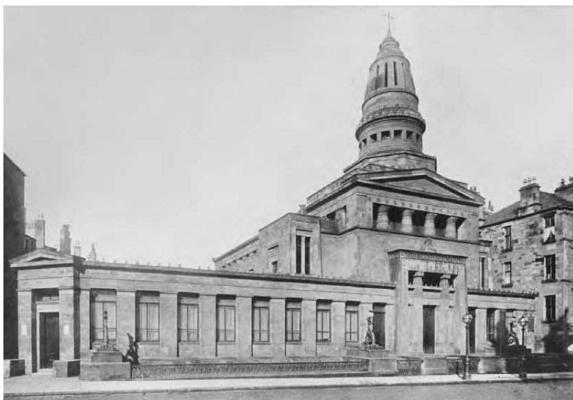
Plate 202 Queen's Park church, Glasgow, of 1867, designed by Alexander 'Greek' Thomson. Both the clerestory of the main temple-block and the long, low, single-storey element at the front have variants of the mullion-columns derived from the Schauspielhaus in Berlin by Karl Friedrich Schinkel of 1818–21. There is a large entrance-pylon with Egyptianising columns set in antis, and two smaller pylons framing variants on the Thrasyllus monument flank the main temple. Four squat Egyptianising columns are set within a frame under the low Greek pediment. The crowning cupola combines Greek, Egyptianising, and almost Indianising elements. Photograph by Bryan & Shear Ltd, Glasgow (Mitchell Library, Glasgow, M 3395 7).
